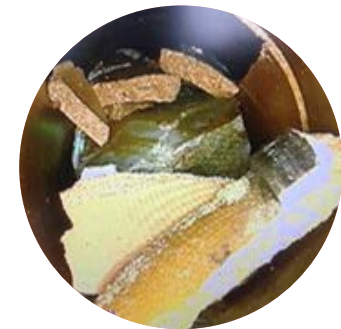
COLLAPSED PIPELINE
