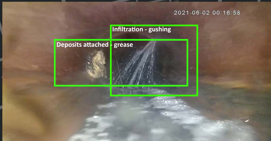
AI AUTOMATIC DETECTED DEFECTS
