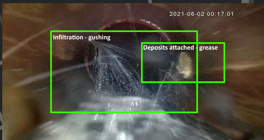
AI AUTOMATIC DETECTED DEFECTS
