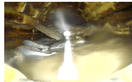
WJ180 REMOVING CONCRETE
