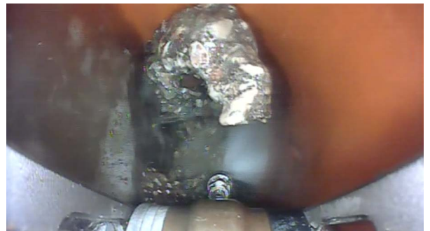
UHP CONCRETE REMOVAL
