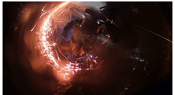
CUTTING A CAST IRON TAP
