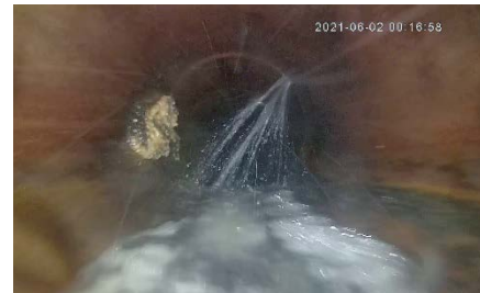
WATER INFILTRATION
