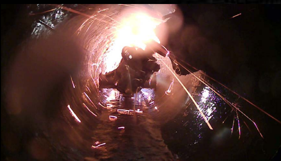
CUTTING A CAST IRON TAP
