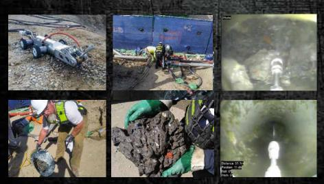
Concrete slurry with aggregate was poured into 250mm, 375mm and 450mm (10", 15", 18") sewer mainlines after boring into an unmarked sewer line during ground stabilization work in a coastal condo development near Los Angeles. The solid obstructions were blocking the sewage flow from a nearby residential area towards the treatment plant and threatening the progress of the construction project.
