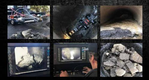
Limescale, the crystallized mineral deposits often found in sewer pipelines of hard water areas, has been successfully removed from multiple sewer pipelines in the Swiss Alps with the Sewer Robotics system.
