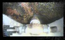
The WJ125 utilizing 1000 bar (14,500psi) to remove tuberculation from this 300mm (12") pipe, as if it was butter.
