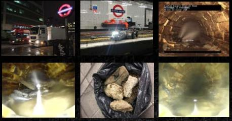
The Sewer Robotics mobile cable reel and control unit were successfully used to remove over 5m (15ft) of concrete from an antique 500mm (20") brick storm water pipeline inside one of London's oldest subway stations.
