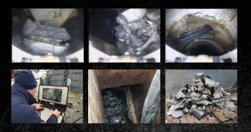
After various failed attempts of different nozzles and cutters, Sewer Robotics was invited to remove the concrete that has been blocking this 400mm (16") sewer main line for the past 10 years.
