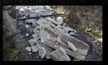
The calcium in this coated VCP 300mm (12") sewer pipe blocked more than half of the pipe and was broken into smaller pieces with the WJ180 at 1000bar (7,250psi).
