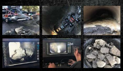
Limescale, the crystallized mineral deposits often found in sewer pipelines of hard water areas, has been successfully removed from multiple sewer pipelines in the Swiss Alps with the Sewer Robotics system.
