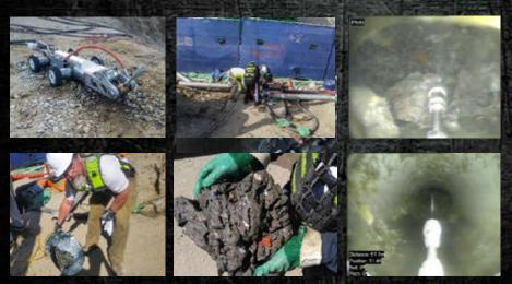
Concrete slurry with aggregate was poured into 250mm, 375mm and 450mm (10", 15", 18") sewer mainlines after boring into an unmarked sewer line during ground stabilization work in a coastal condo development near Los Angeles. The solid obstructions were blocking the sewage flow from a nearby residential area towards the treatment plant and threatening the progress of the construction project.
